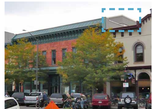
Rooftop addition where the setback distance was required to equal the height of the new addition.
