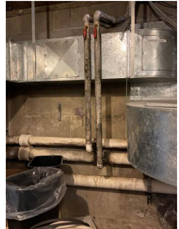
Cafeteria HVAC room: discoloration on pipe
