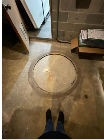
Cafeteria HVAC room. Old sewer line access hatch. Maintenance believes its bypassed but could still hold water leading to high humidity in room.
