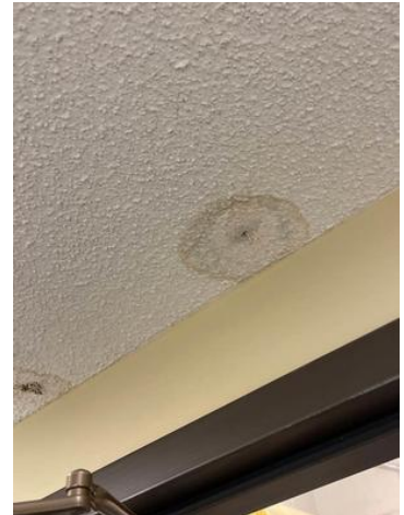
Library: discoloration and staining on ceiling outside of the small storage room.
