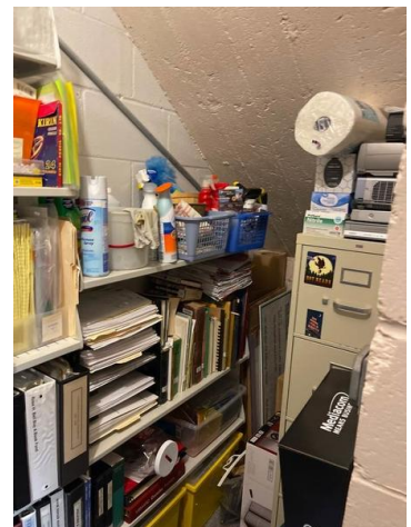
Library small storage room. Non vented door and no HVAC in this area. Very damp and mildew odor.
