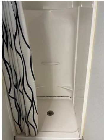
Showers in lower shower room. Discoloration on grout; assumed visible fungal growth
