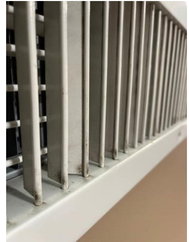
Cafeteria air supply grate discoloration
