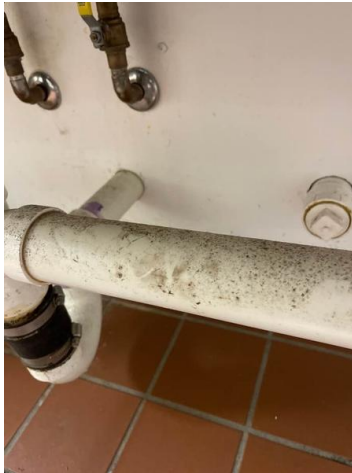
Kitchen. Discoloration, assumed visible fungal growth
