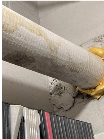
Library small storage room. Discoloration at wall and on pipe insulation.
