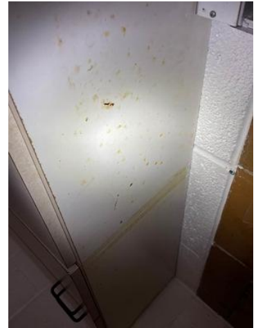
Gymnasium concessions area. Bottom of metal cabinets rusting from excess moisture
