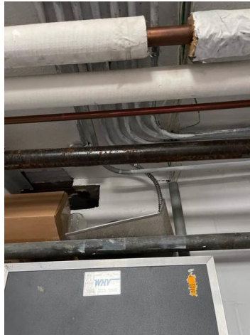
Boiler room. Non insulated pipe. Maintenance noted on certain days this pipe just drips directly on to floor.
