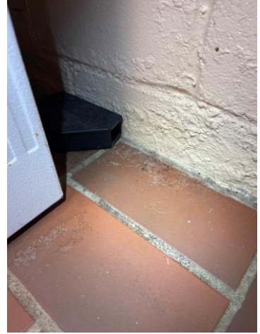
Kitchen. Efflorescence on block wall. Discoloration, assumed visible fungal growth
