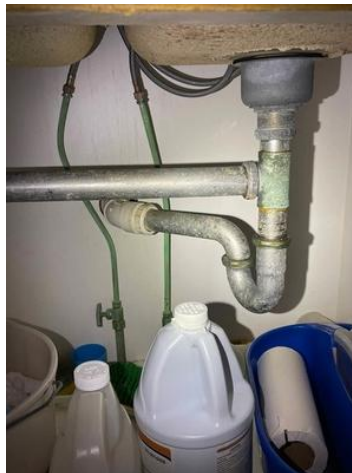
Gymnasium concessions under sink. Excessive moisture evident in the past. Growth on metal pipes
