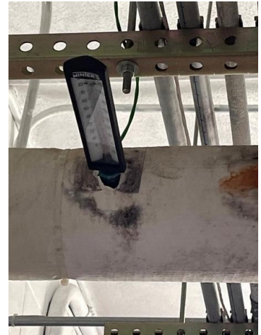
Boiler room: discoloration on pipe insulation
