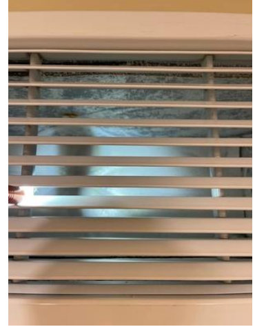
Library return air duct painted interior insulation. Discoloration may be present.
